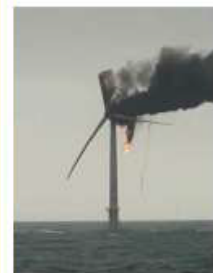
▲ The Arklow Bank turbine shortly after the suspected lightning strike. (Photo: John Morgan)
